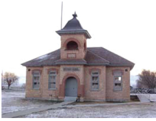
Fairfield School House, 1898
