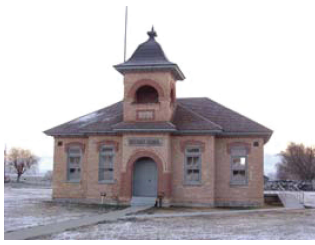
Fairfield School House, 1898
